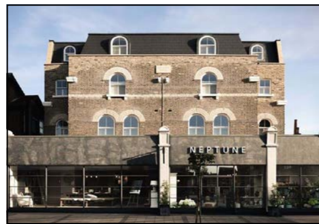
Fig. 166: Vertical extension to Neptune House in Merton (TBC)
