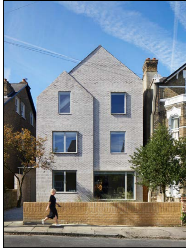
Fig. 187: Vertical extension and re-cladding of an existing house following the principles of Street Infill development. Designed by Alma-nac (website: www.alma-nac.com, photography: TBC)
