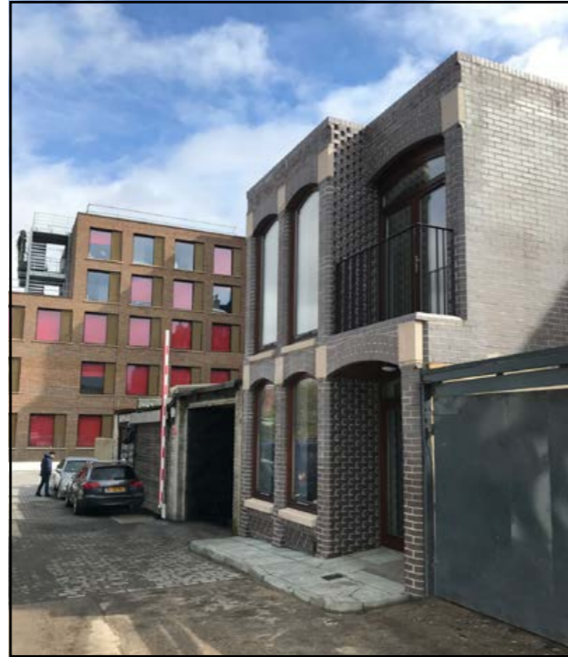
Fig. 184: New mews house in New Cross designed by Kennedy Twaddle (website: www.kennedytwaddle.com , photography: Chris Twaddle)
