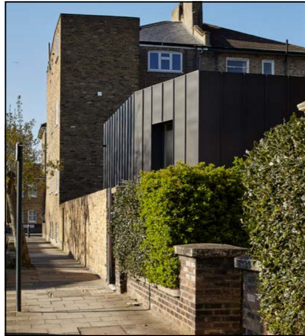
Fig. 144: This scheme by Tectonics Architects achieves a certified Passivhaus home on a small side-facing site in Hackney. (website: www.tectonics-architects.com , photography: Alex Sarginson)
