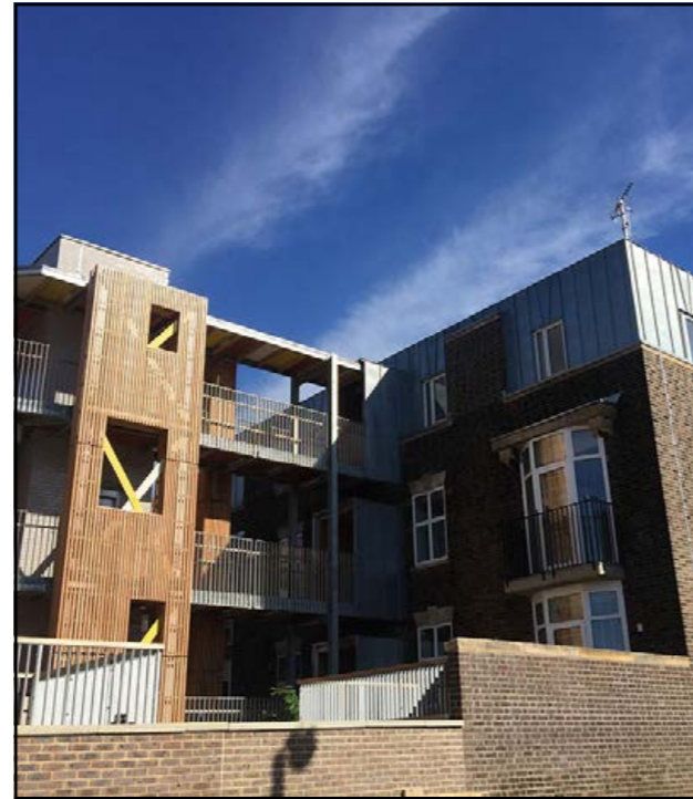
Fig. 160: The refurbishment and vertical extension of St Paul's House in Deptford by Ash Sakula (website: www.ashsak.com , photography: Ash Sakula)
