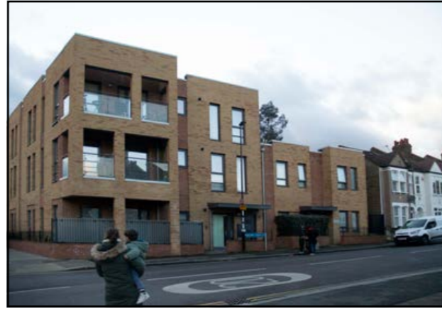
Fig. 134: Corner Development in Sydenham
