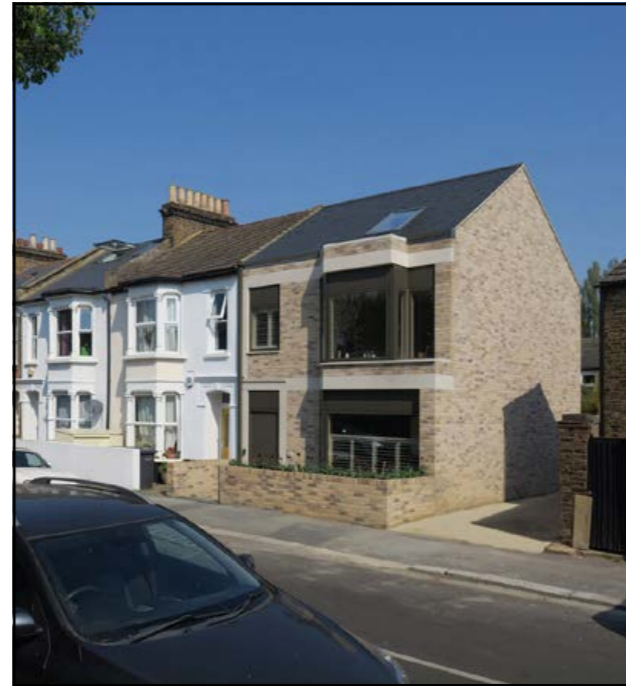
Fig. 118: Replacing disused garages, House on the End by architect 1200 Works extends an existing Victorian terrace to create a new family home. (website: www.1200works.com, photography: TBC)
