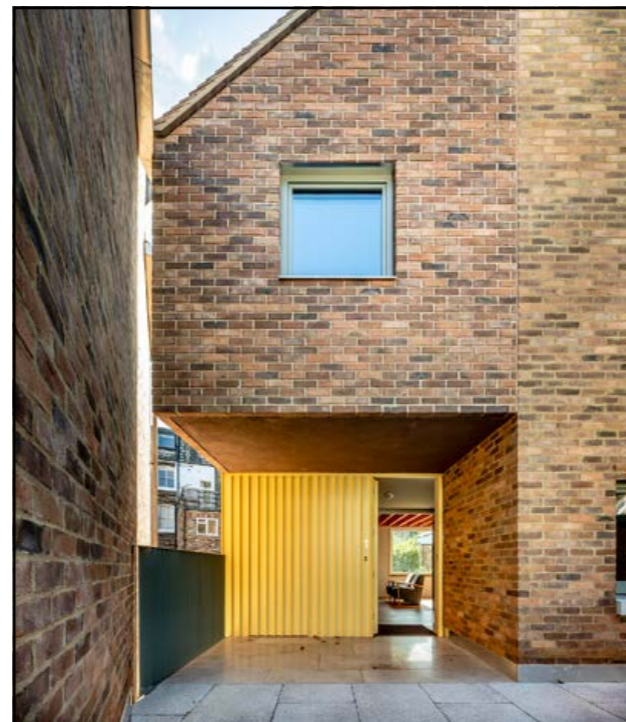
Fig. 171: Moore Park Road in Hammersmith is a backland development designed by Stephen Taylor Architects (website: www.stephentaylorarchitects.co.uk , photography: TBC)
