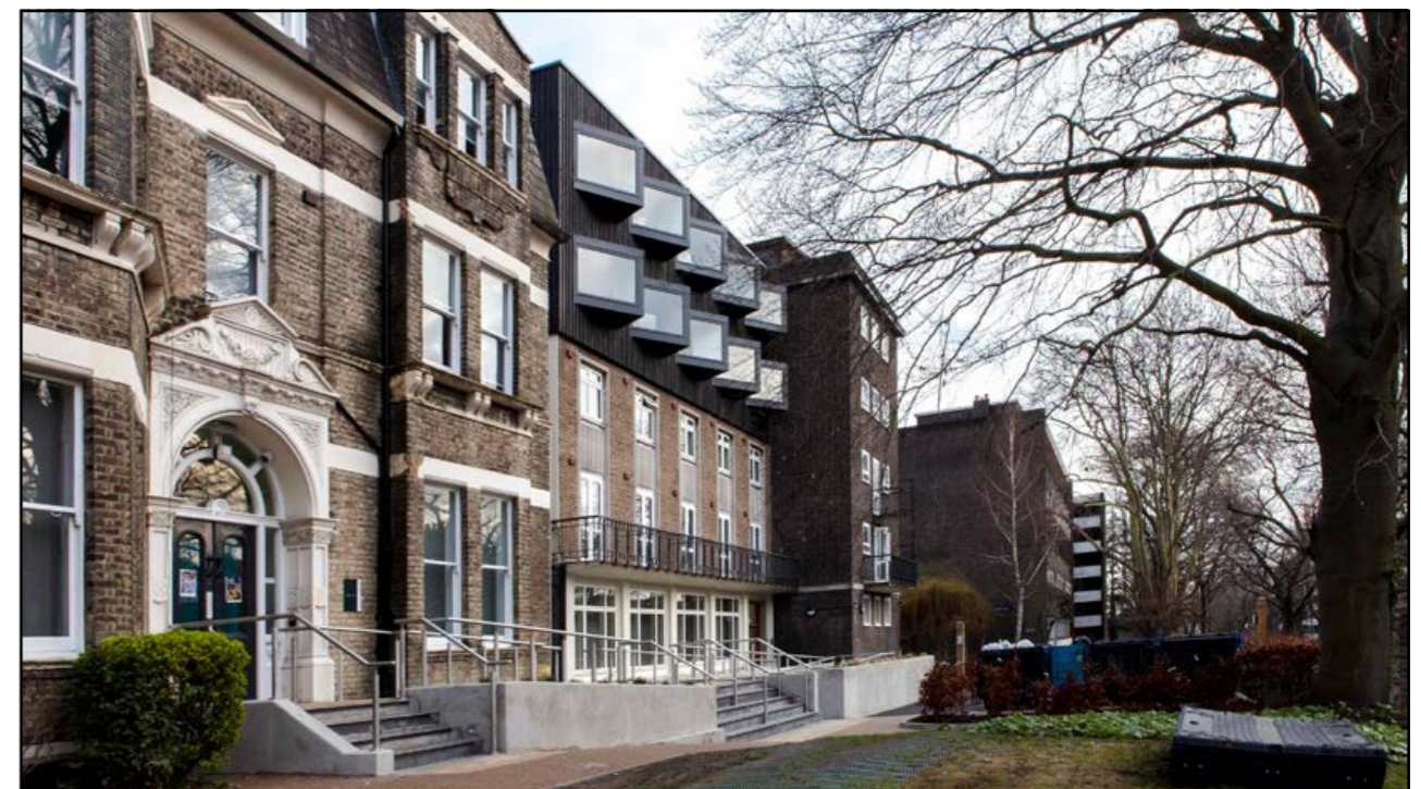
Fig. 159: Extension to Raymont Hall by Hawkins\Brown providing new student accommodation. (website: www.hawkinsbrown.com , photography: Francesco Montaguti)
