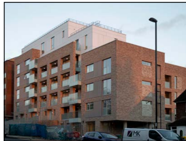
Fig. 103: Forster House in Whitefoot designed by Levitt Bernstein Architects (Website: www.levittbernstein.co.uk, Photography: RCKa)
