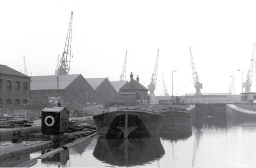
Fig.11 Timber Wharf in Operation (1970's)
