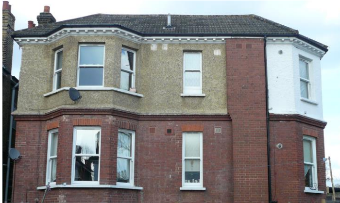
Image 71: Removal of chimney stacks can make a house appear truncated.
