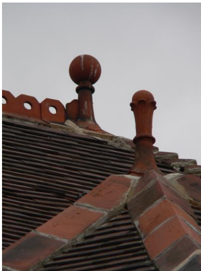
Images 50 and 51: Terminations are marked by finial tiles in ball or hook designs.
