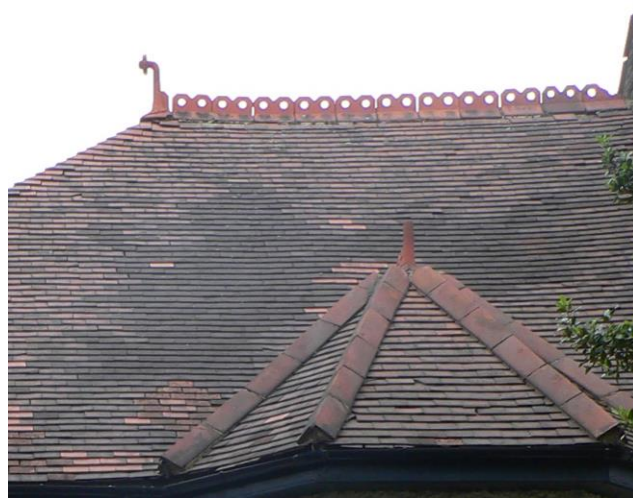
Images 50 and 51: Terminations are marked by finial tiles in ball or hook designs.
