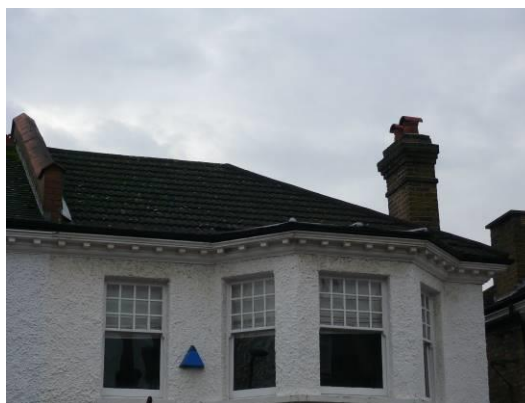
Images 62 and 63: Replacement of roof covering with non-traditional materials can detract from the appearance of the property
