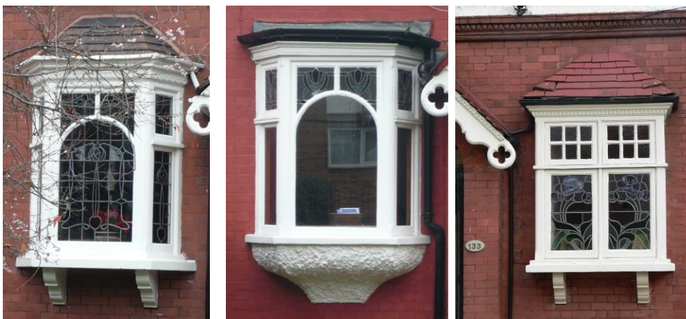
Images 44 and 45: Oriel windows come in four variants: those supported on brackets (left), those supported on a rough cast corbel (middle), those with an arched lower light and those with flat topped lower lights (right).
