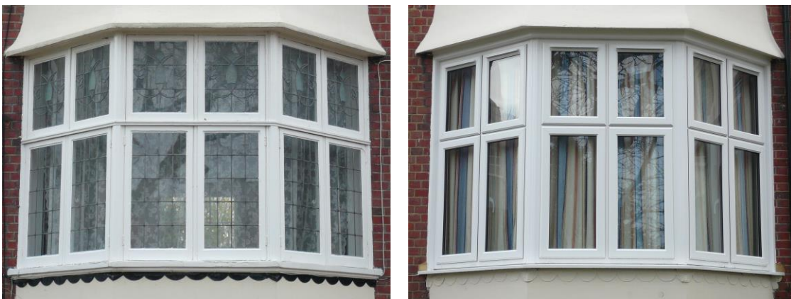
Image 66 and 67: The image to the left shows the historic stained glass with leaded panes and the image to the right the loss of the feature and heavy profile of the window.
