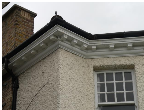
Image 36: Rough cast is a common material used on first floor elevations.
