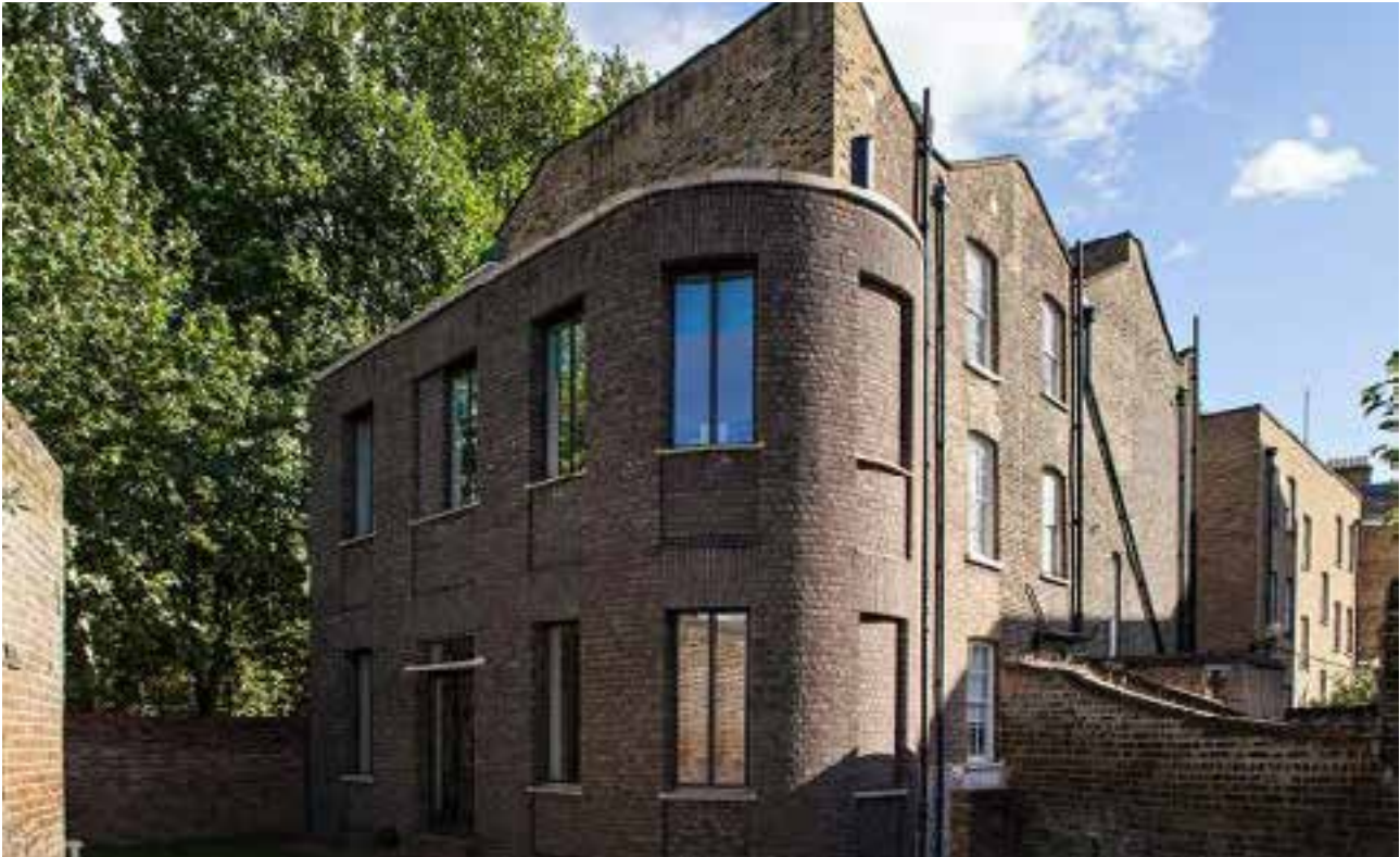
Fig. 203: Although a side extension, this development illustrates many aspects of best practice that should be applied to proposals for rear extensions in the Conservation Area. It is clearly subservient to the host historic building, so that the roof and other significant details of the host building can be seen clearly. Materials and proportions are inspired by the historic building, with the result that the extension sits comfortably against it.
