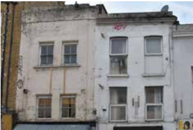
Fig. 199: Traditional timber sash windows (left) alongside replacement uPVC windows (right)
