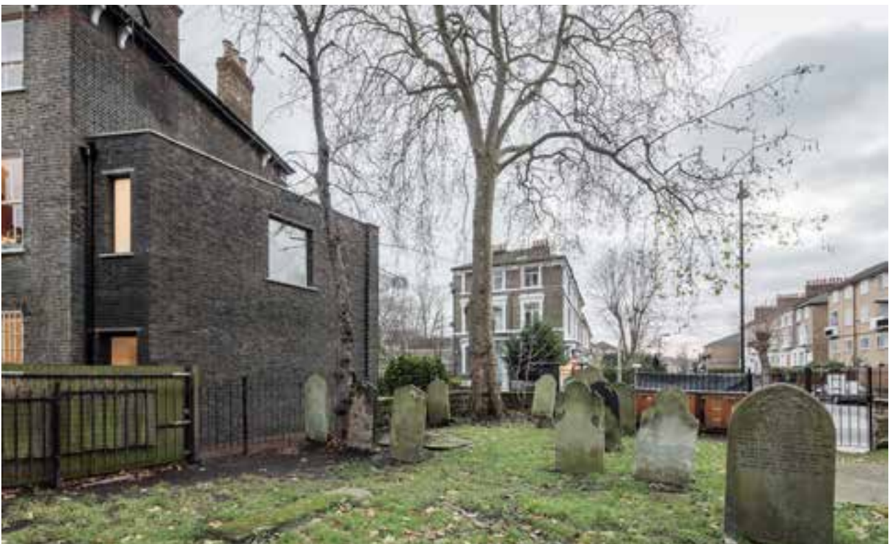
Fig. 204: Another example of good practice. This is clearly an ancillary extension, and has carefully matched brickwork and subtle detailing.
