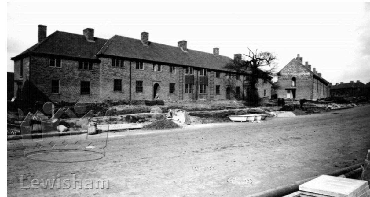
Ongoing construction work on the Bellingham Estate in 1923. The houses have been completed but baths are outside waiting to be plumbed in and the road is still unmade. Source: Borough Photos
